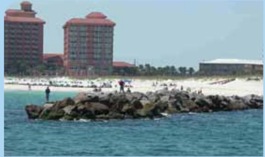
Figure 6.5. Jetties are designed to reduce erosion, but in some cases, have the opposite effect by disrupting the natural movement of sand, leading to surpluses or deficits of sand along a beach.
