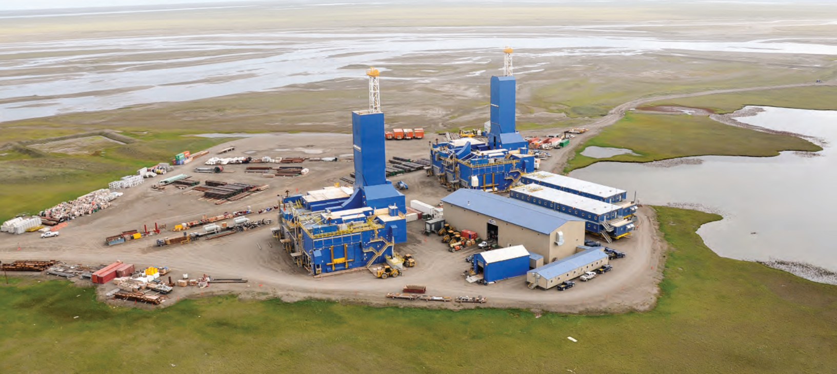
Oil field support facility at Prudhoe Bay (credit: M. Lindeberg, National Marine Fisheries Service/NOAA)
