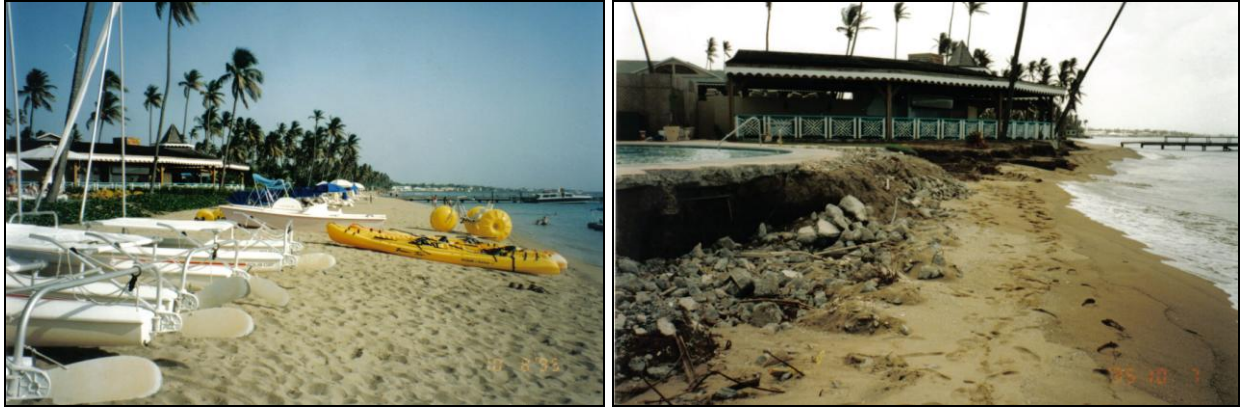
In the absence of construction setbacks, beachfront property is highly vulnerable to damage from natural erosion and storm cycles, as illustrated by this Four Seasons Hotel in Nevis, pictured before and after Hurricane Luis. Photos: Gillian Cambers (UNDP).
