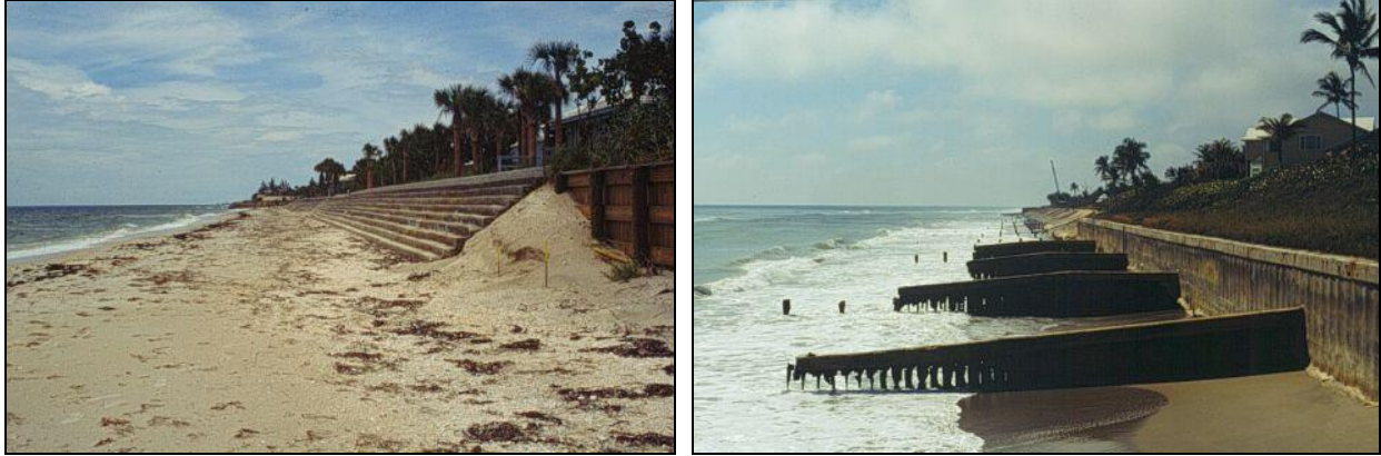
Beach armoring, such as this seawall (left), can worsen localized erosion and reduce sea turtle nesting habitat, while jetties (right) disrupt longshore sand transport and starve down-current beach segments, also reducing sea turtle nesting habitat (photos: Florida Fish and Wildlife Research Institute, http://research.myfwc.com/gallery/ ).
